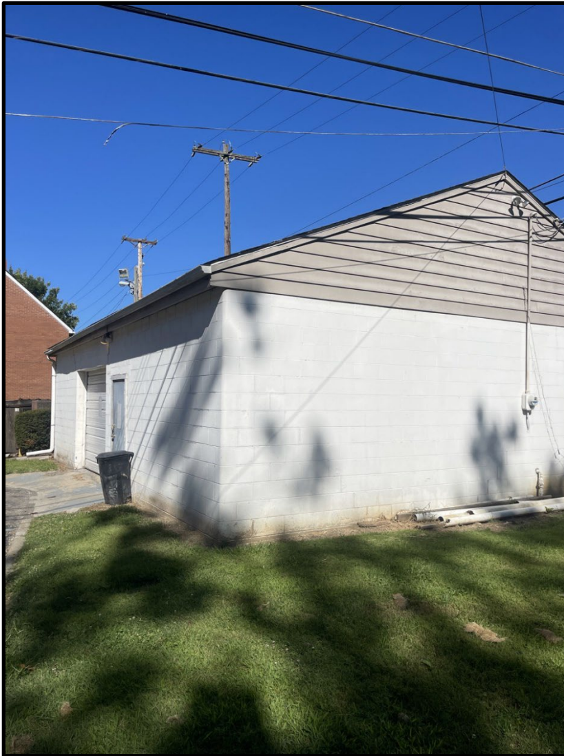
31. View of existing maintenance shed to be demolished, looking northwest.
