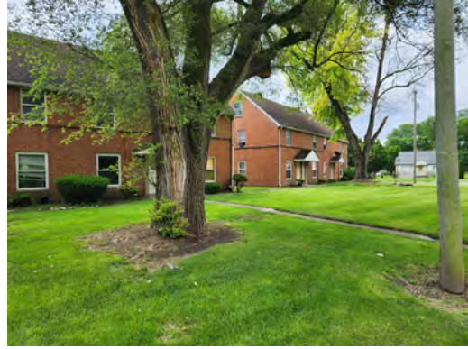
PHOTO #2 WEST ELEVATION
