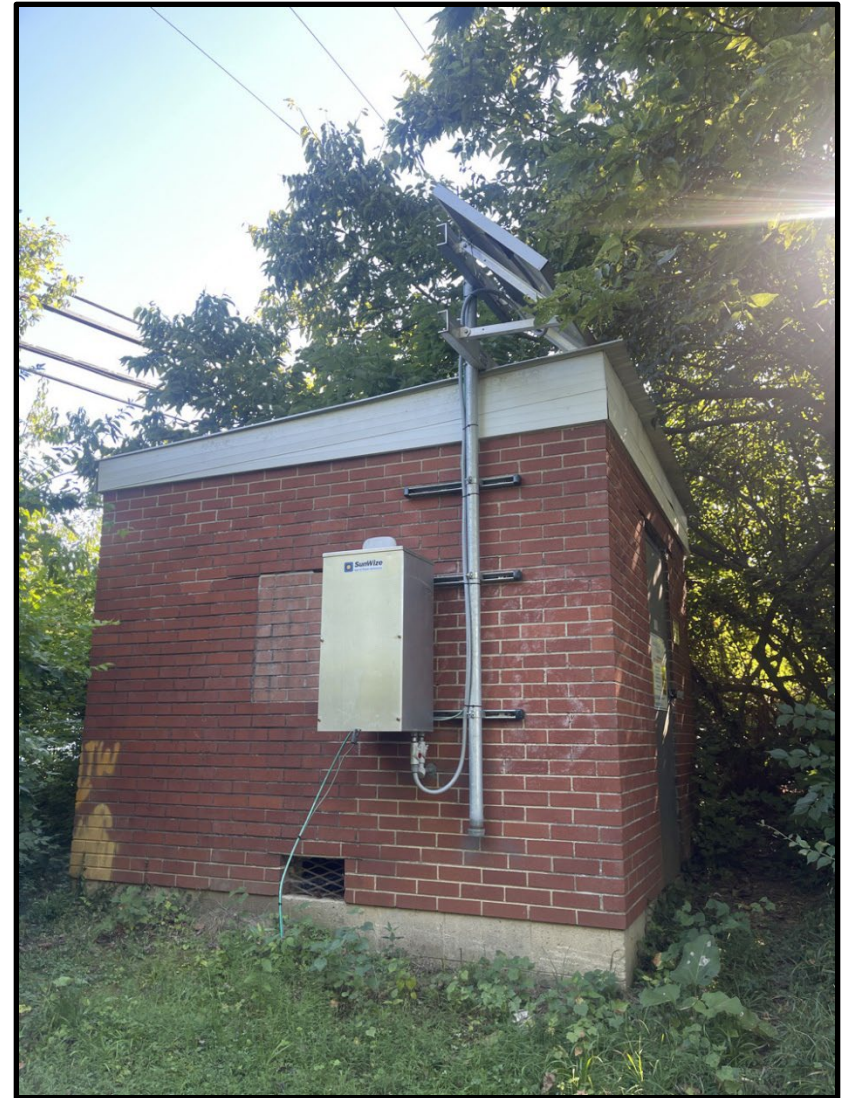
6. View of Columbia Gas building located on the northwest portion of the project site, looking northeast.
