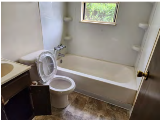
PHOTO #23 RESIDENTIAL UNIT BATHROOM
