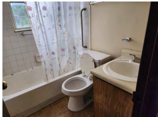
PHOTO #24 RESIDENTIAL UNIT BATHROOM
