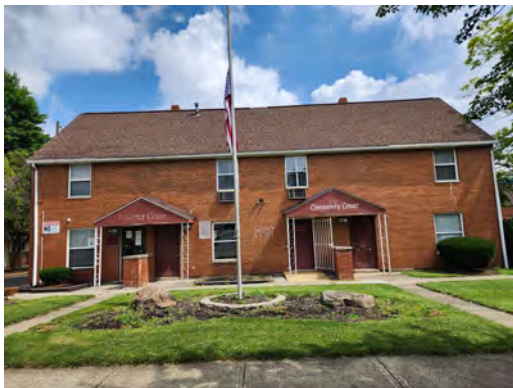
PHOTO #5 SOUTH ELEVATION OFFICE/COMMUNITY BUILDING
