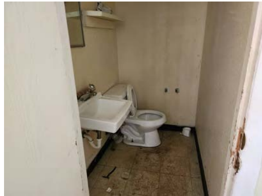
PHOTO #16 LAUNDRY BUILDING BATHROOM
