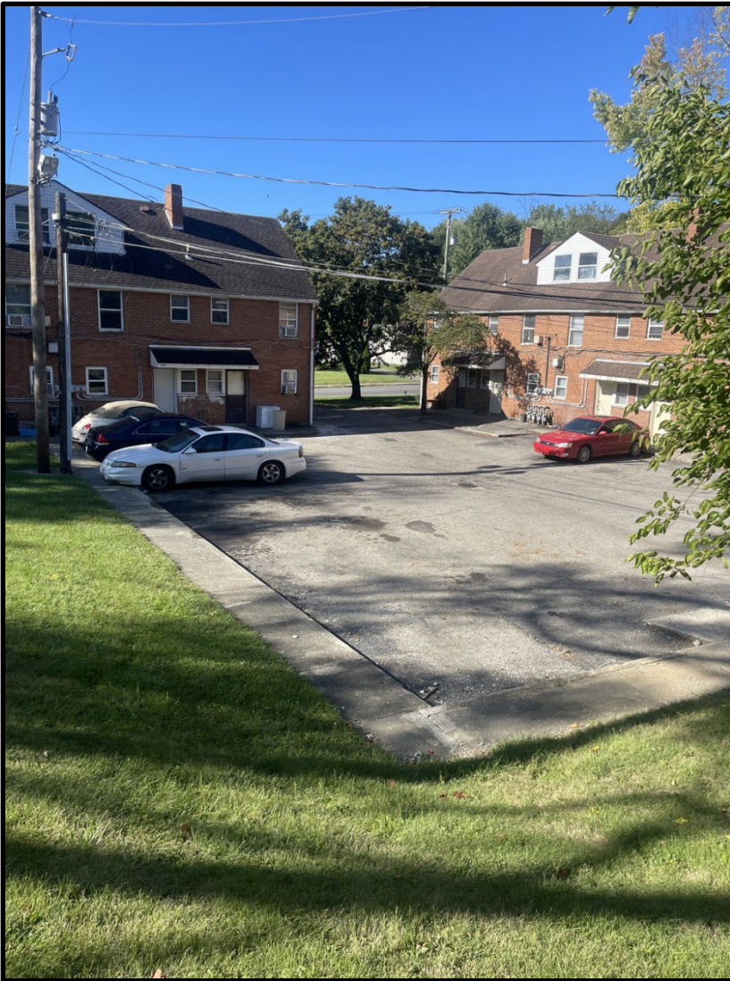
5. View of existing apartment buildings proposed for redevelopment as a community and maintenance building, looking southwest.
