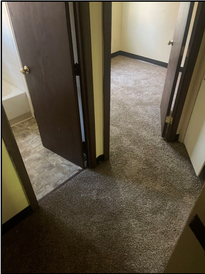
47. Representative view of hallway to bedroom and bathroom at the existing apartment in the project area.
