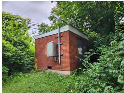
PHOTO #30 NATURAL GAS PIPELINE BUILDING
