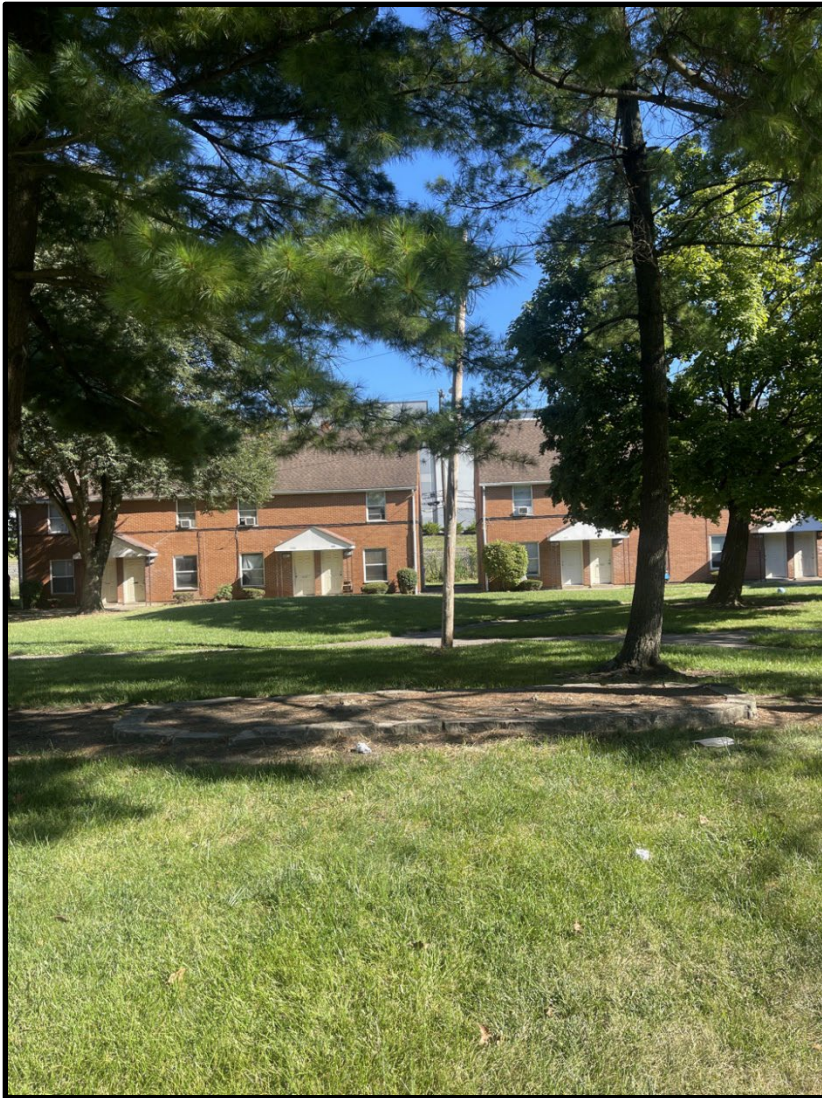
23. View of courtyard between existing apartment buildings within the project site, looking north.
