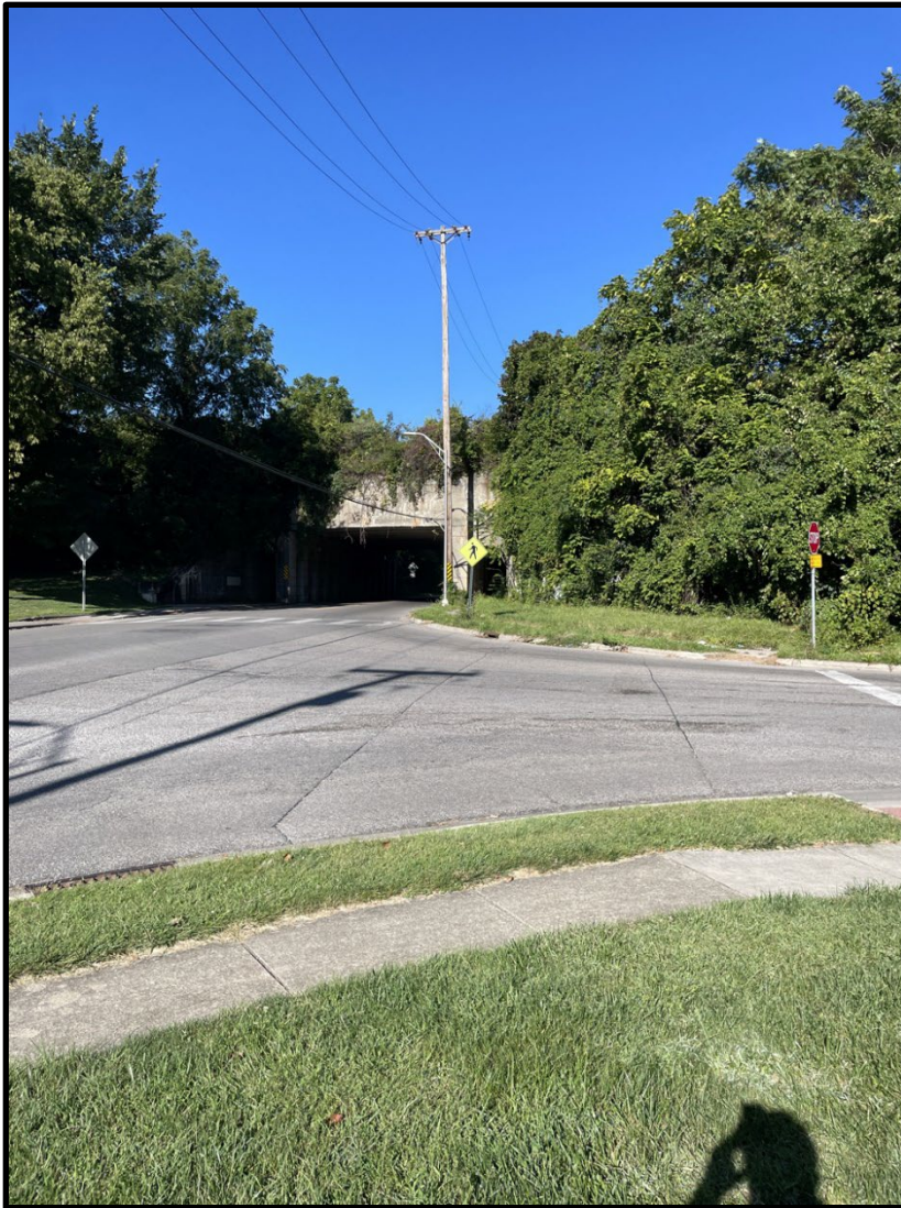
1. View of existing bridge and forested area adjacent to western side of project site along Sunbury Road, looking west.
