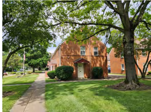
PHOTO #4 EAST ELEVATION OFFICE/COMMUNITY BUILDING
