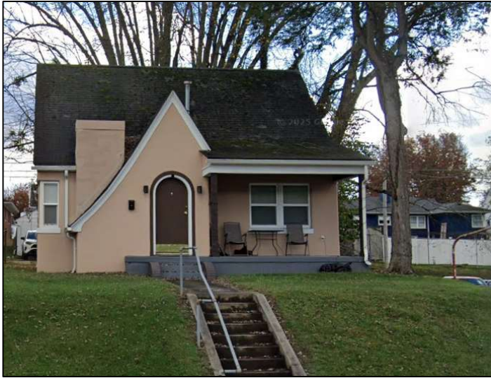
Photo 5: 611 3 rd Avenue, facing south.
