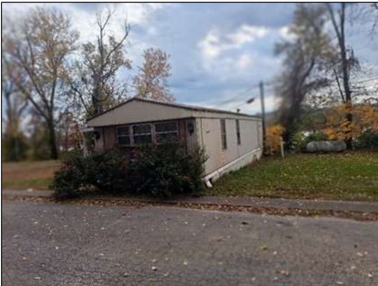
Photo 27: Remaining mobile home in Project Area, facing southeast.
