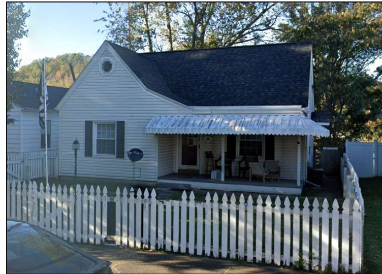
Photo 12: 622 2 nd Avenue, facing northwest.
