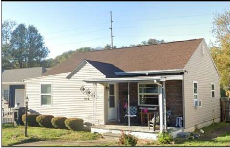
Photo 9: 616 2 nd Avenue, facing northwest.
