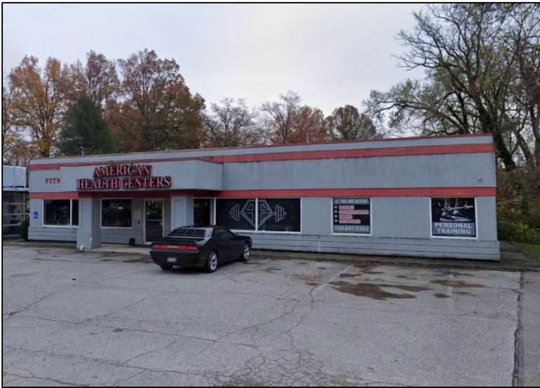
Photo 1: 733 3rd Avenue, facing south.
