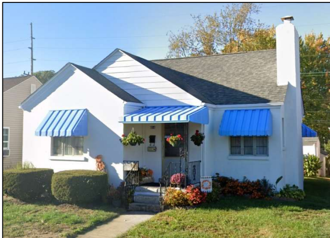
Photo 7: 614 2 nd Avenue, facing northwest.
