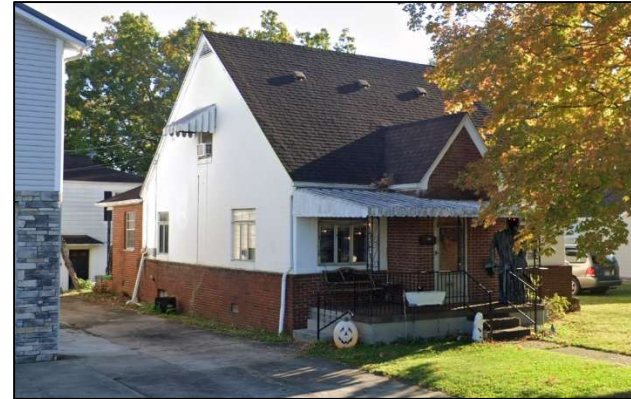
Photo 10: 619 2 nd Avenue, facing south.
